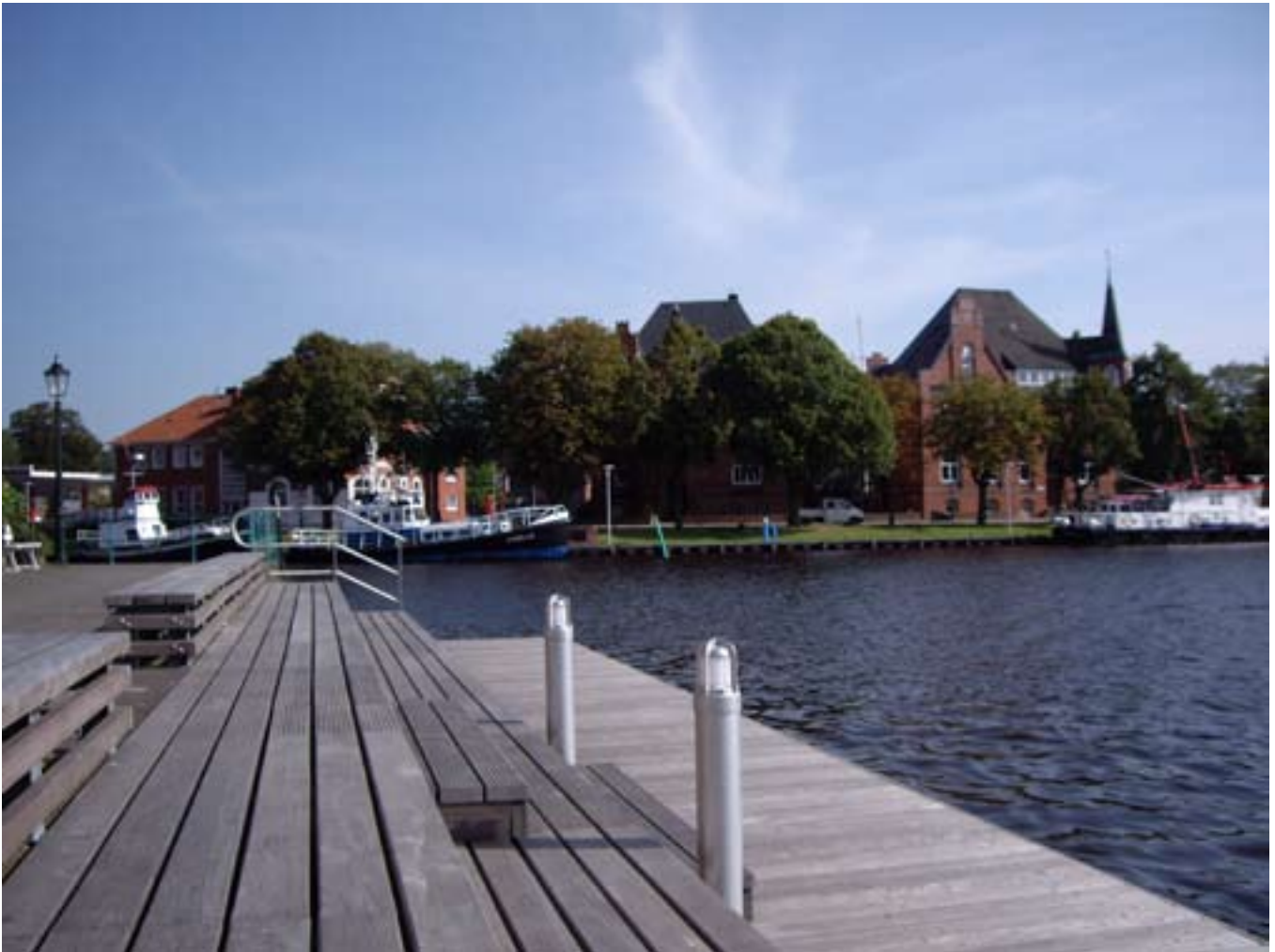
Interreg III B North Sea Programme: Project Watercity International II at Emden, Stigt Schreyershoek (wooden stairs)
